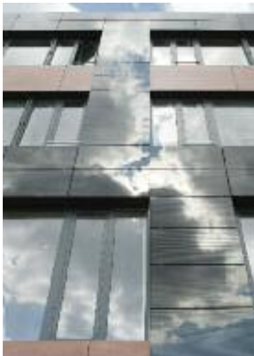
Building integrated photovoltaics: a thin film panel in a façade-integration. © Goldbeck solar GmbH/Sulfurcell
