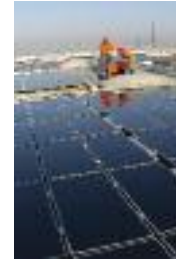
Workers installing thin film modules on a flat roof. © First Solar
