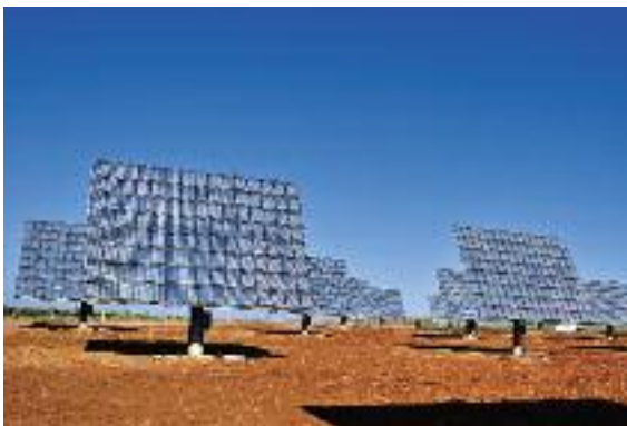
Concentrator Photovoltaics installed on trackers to follow the sun. © Concentrix
